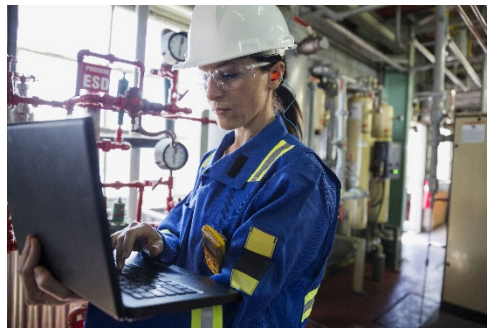
Oil & gas facility
